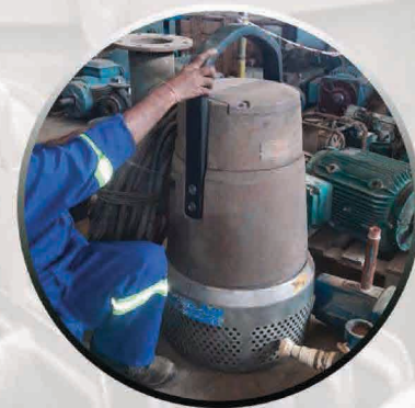
Submersible Pump Repairing
