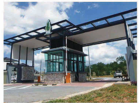
Entry Exit Gate Canopy
