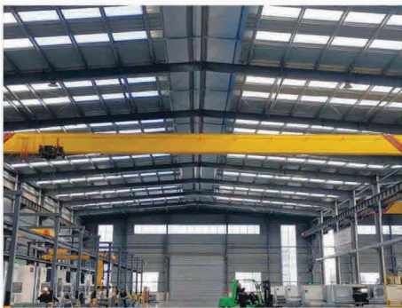
Fabrication Workshops with Crane
